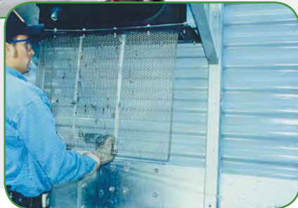
Inlet strainer inspection for Series 3000
